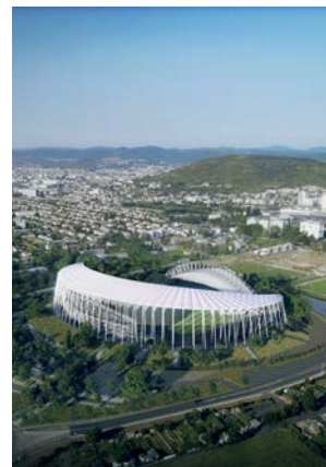
© ATELIER FERRET ARCHITECTURES
